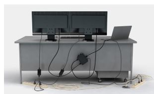
Conventional solution Messy cabling
